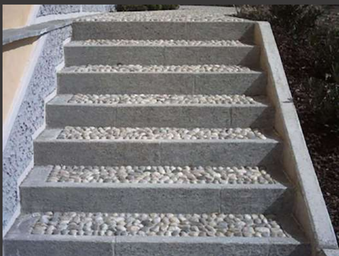
ALZATE IN GRANITO SCALE IN CIOTTOLI
